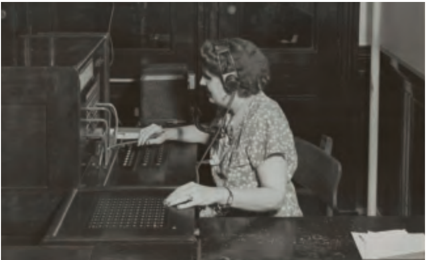
Early switchboard operations.
